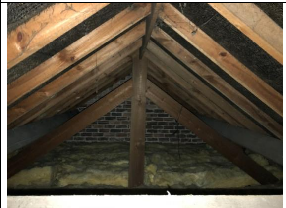
Photo 13: Loft void western aspect
