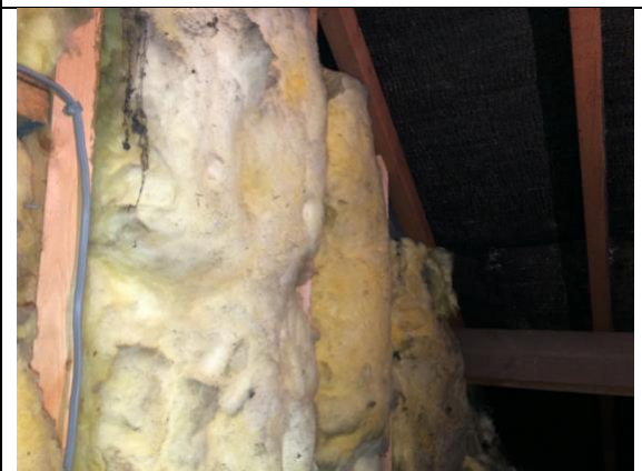
Photo 12: Loft void showing the wall insulation of the loft conversion
