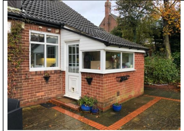
Photo 4: Porch on the rear aspect
