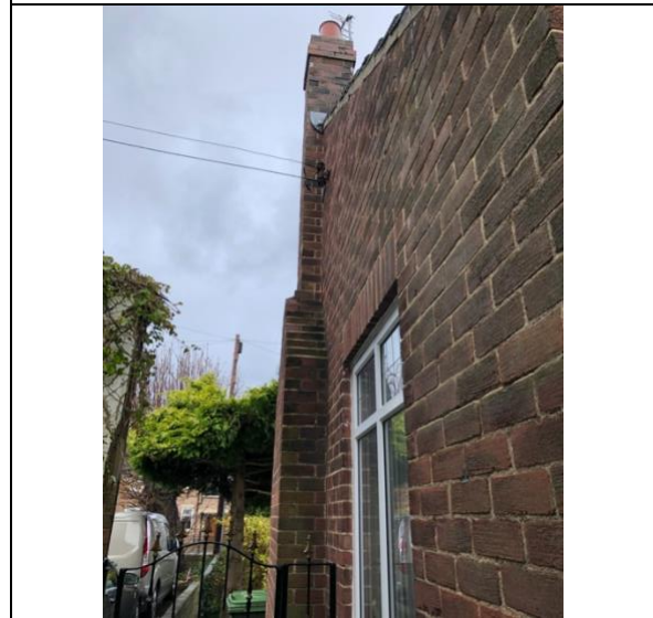
Photo 5: Southern gable end
