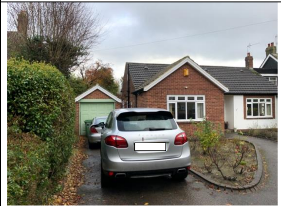
Photo 2: Front aspect & garage (northwest)
