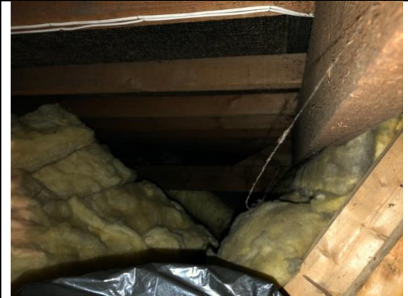
Photo 11c: Loft void along edge of the loft conversion. Not inspected fully.
